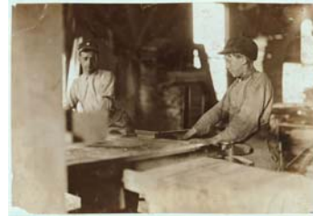
Boy Working at the Saw, N. Y. Dimension Supply Co., Evansville , Ind. Location: Evansville, Indiana.
