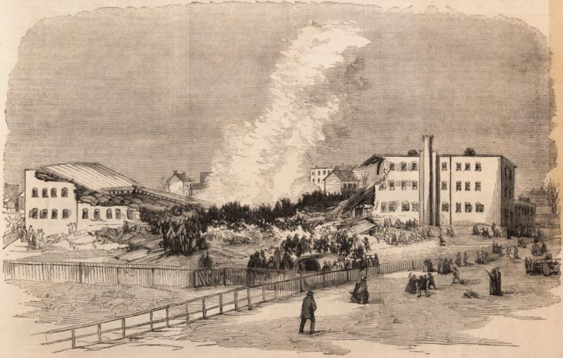
RUINS OF MESSRS. AMES & MOULTON'S FACTORY, WILLIAMSBURG, DESTROYED BY STEAM-BOILER EXPLOSION, ON FRIDAY MORNING, FEB. 2, 1860.—(SEE PAGE 197.)
