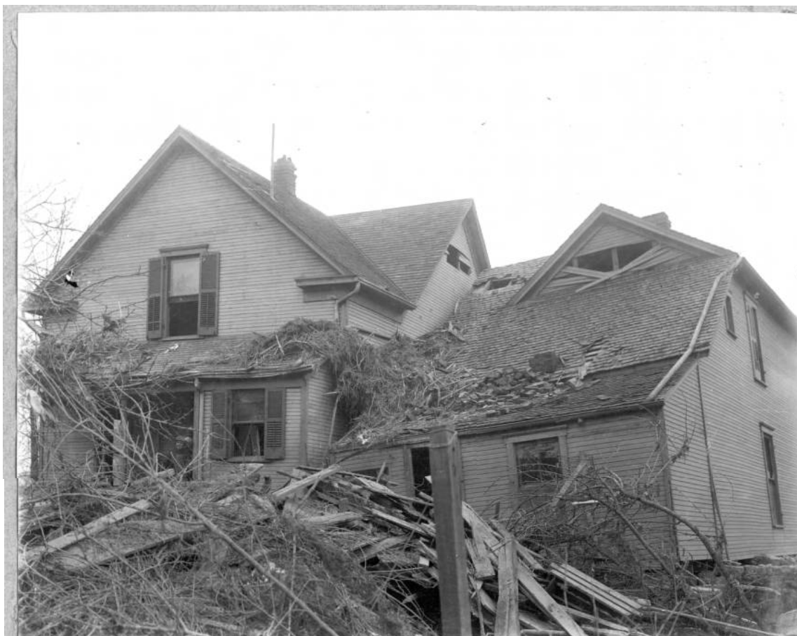
People trapped in the upper stories of their homes chopped holes in the attic walls and roofs in order to escape.
